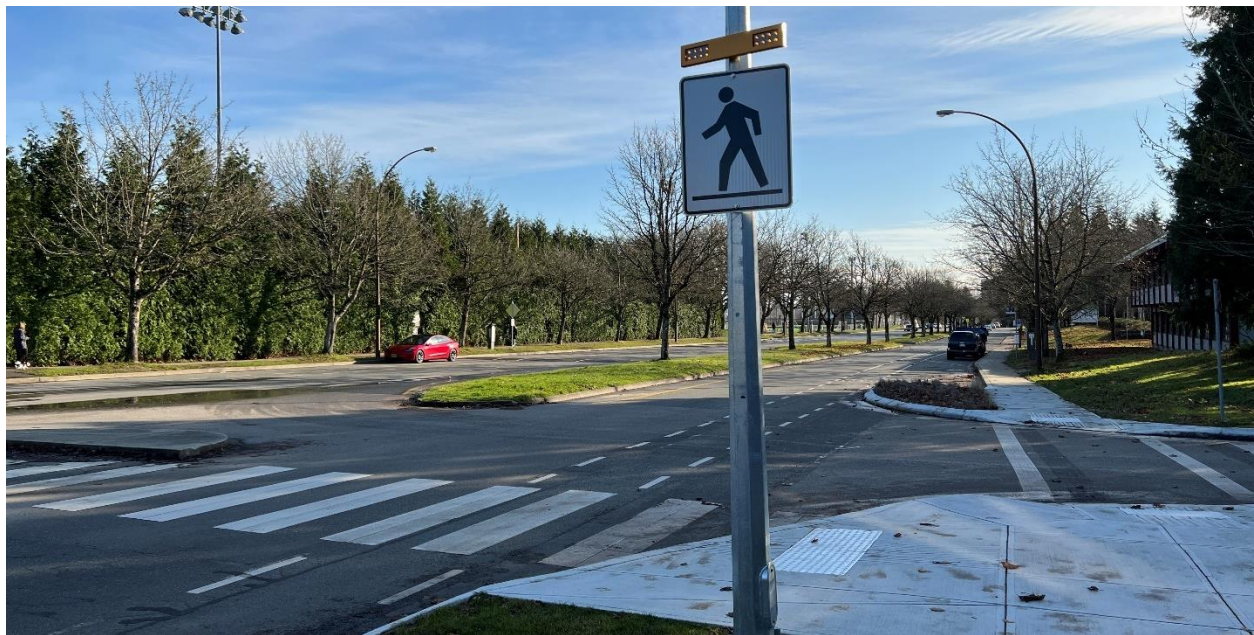
Figure 17 – Additional Pedestrian Controlled Traffic Lights and Sign
