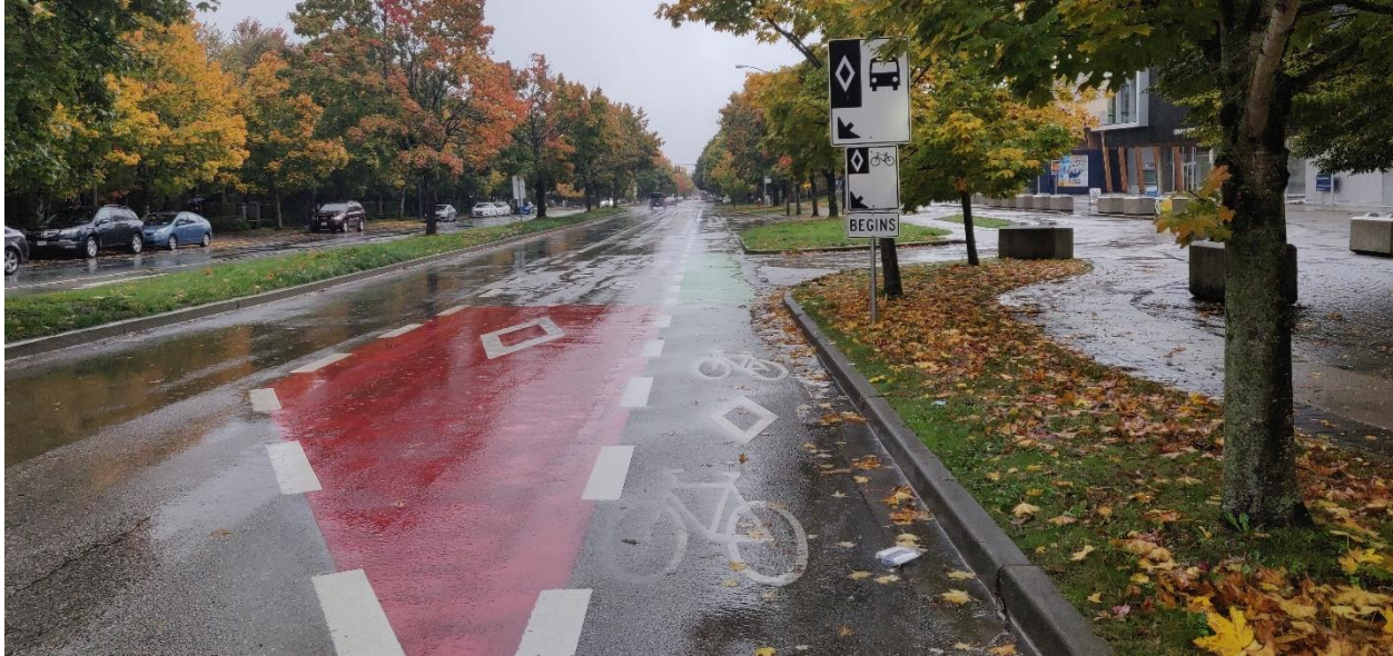
Figure 7 – Existing Southbound Lane Configuration
