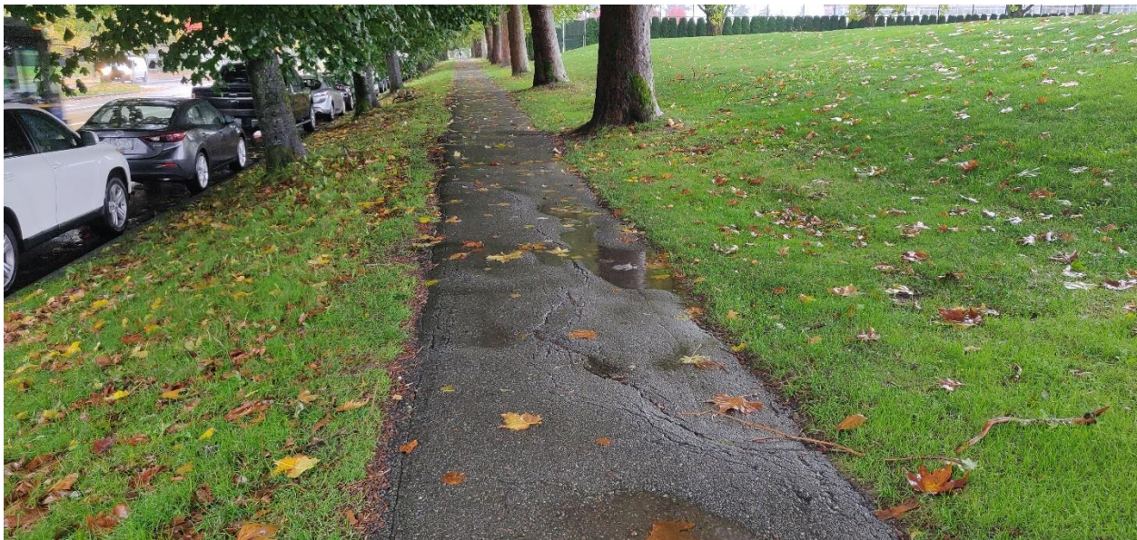
Figure 10 – Existing Southbound Sidewalk (Near Sporting Fields)
