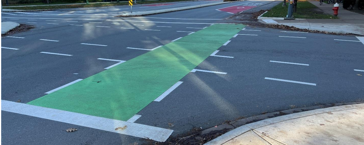
Figure 18 – High Visibility Traffic Markings for Cyclists Crossings
