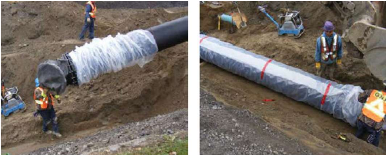
FIGURE 20: POLYETHYLENE WRAPPING AROUND DUCTILE IRON PIPE (DIPRA, 2016)
