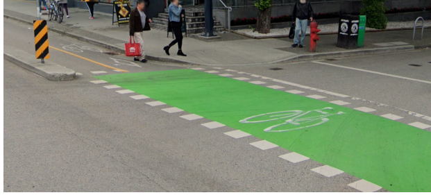
Figure 8: Bicycle crossing with green pavement treatment and elephant's feet markings
