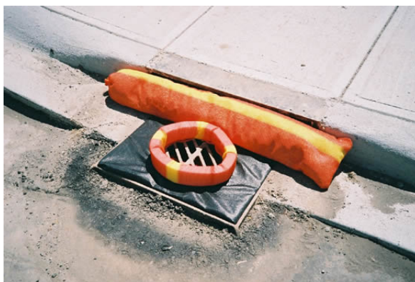
Figure 21: Catch Basin Bags as Shown in Downtown Vancouver. (Source: Photographed by Carlson Lau)
