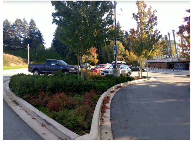
S2: Parking lot at Thunderbird Stadium - Existing bioswale system to manage runoffs
