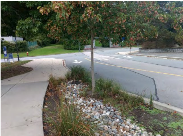
S3: Parking lot entrance at Thunderbird Stadium - Bio-retention trenches along the road side
