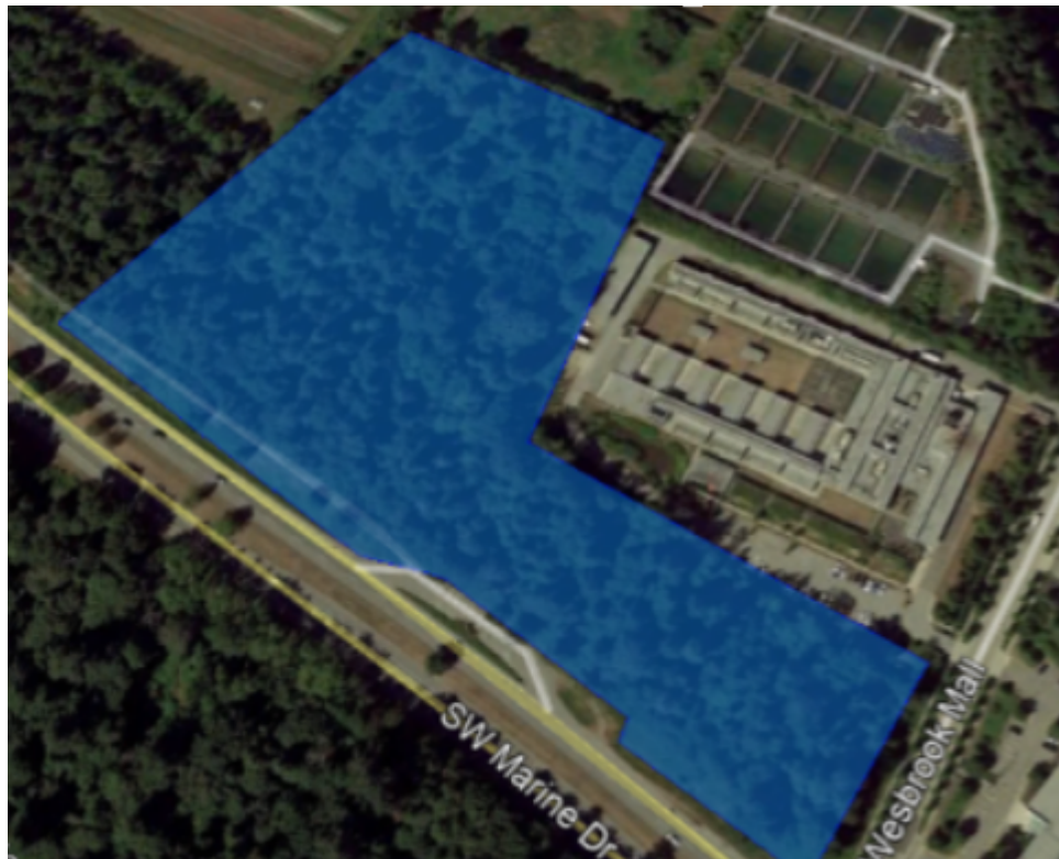
Figure 1: Aerial view of existing site.
