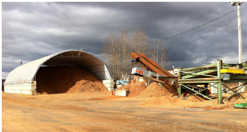
Figure 8. A shed at Cloverdale Fuels Ltd.
