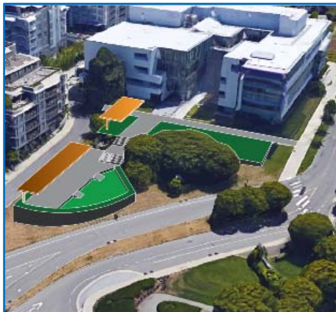
Figure 4: Allard Hall Lookout Terrace
