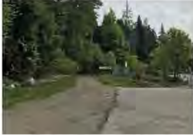
Poor walking conditions in South Campus
