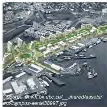
Dockside Green Victoria, BC Master planned community with LEED Platinum target with a closed loop 100% on-site sewage treatment system that uses treated water for flushing toilets, landscape irrigation and water features. Water consumption is 65% lower than conventional developments.
