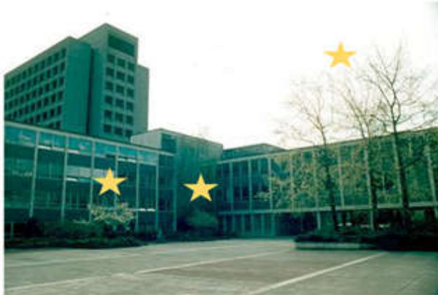
Figure 17. Buchanan West Courtyard looking south. Photo credit: [unknown], 1979.
