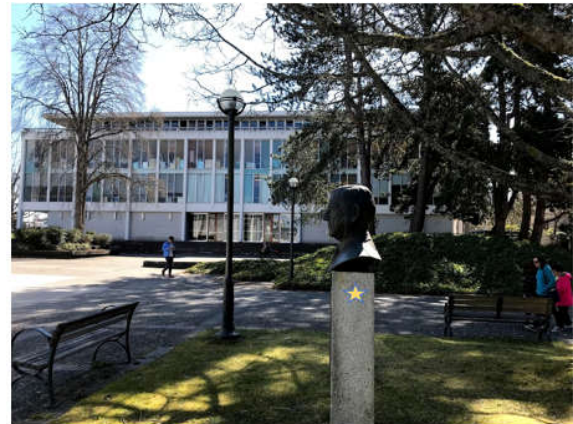
Figure 16. Sunken Plaza looking south. Photo credit: Borschneck, S., 2019.
