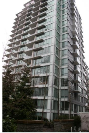
Fig 6. Spandrel glazing used in Academy building to cover the construction material
