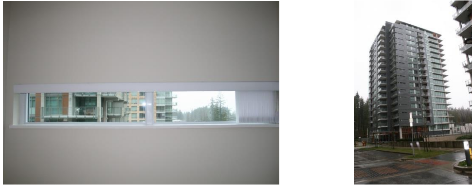
Fig 8. Strip windows on the north and west elevations
