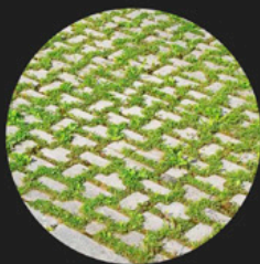
Permeable pavers for parking
