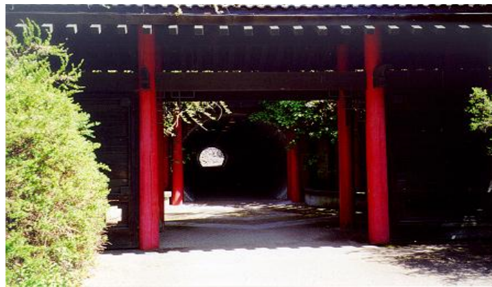
Figure 10: Tunnel West entrance
