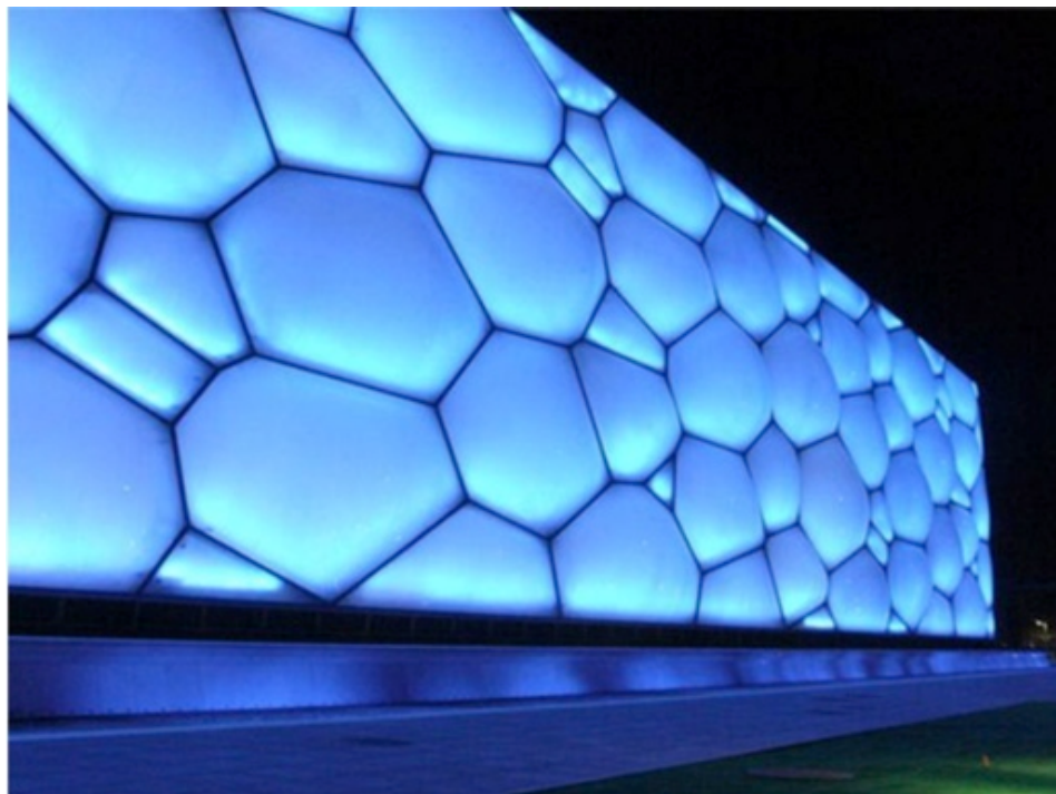
Figure 7 - ETFE Panels at Night (FIXR, 2011)
