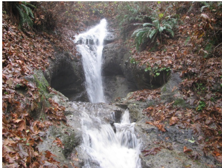
Figure 20 - Trail 7 Outfall Showing Extensive Erosion and Undercutting of Gully Wall
