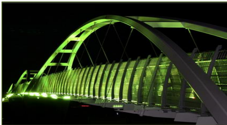
Figure 9: Tynehead Overpass at Night
