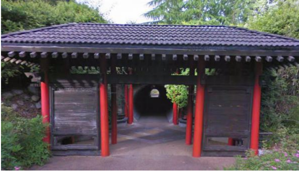
Figure 15: Current Tunnel Connecting the North and South Garden
