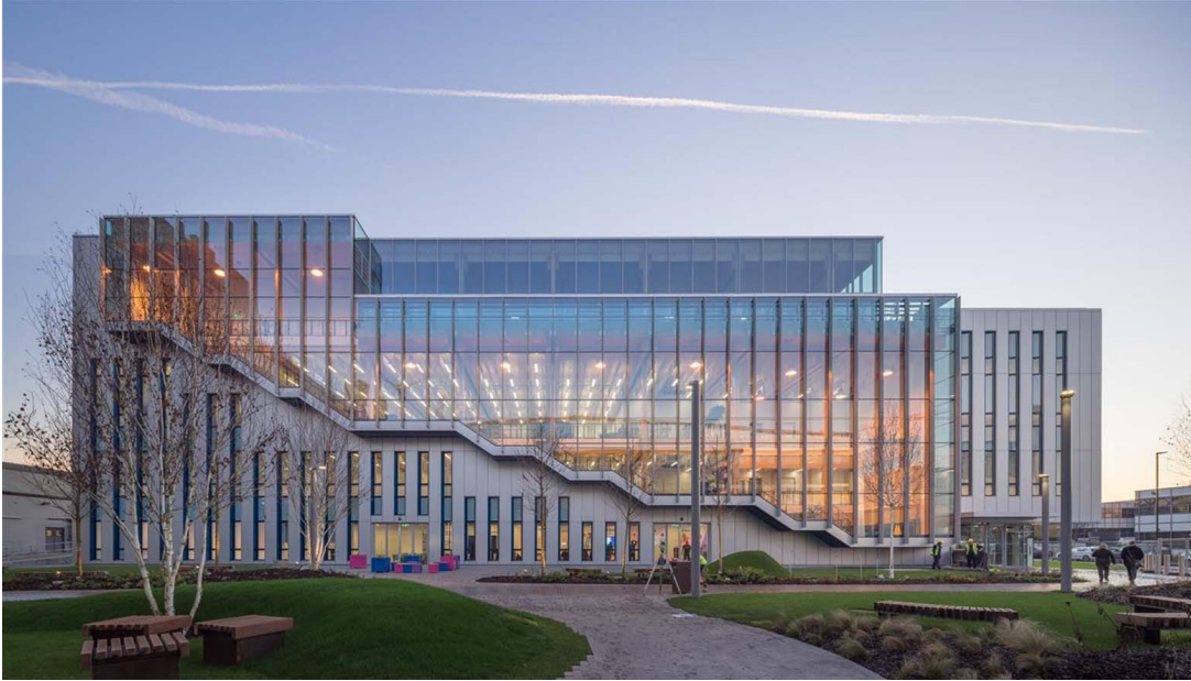
Figure 11 - Photo of Sky's Believe prefabricated building [20]
