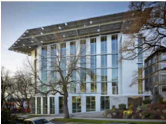
Figure 2 - Rooftop solar system on the multipurpose Bullitt Centre in Seattle, WA [5]
