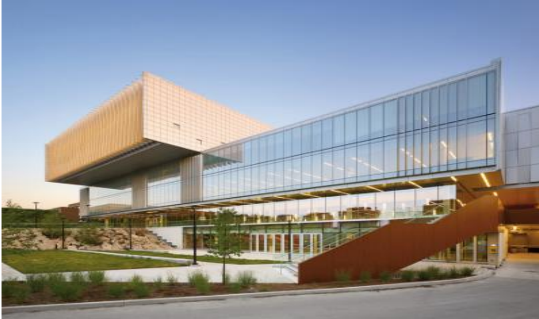
York University - Student Centre: LEED Gold Certification
