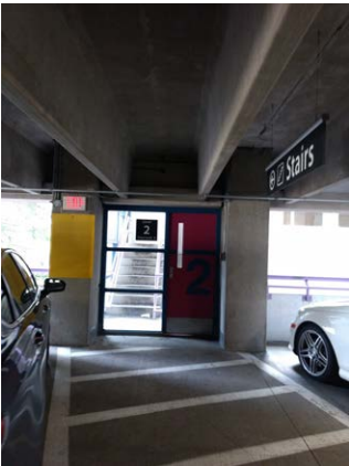
Stairs at each floor
