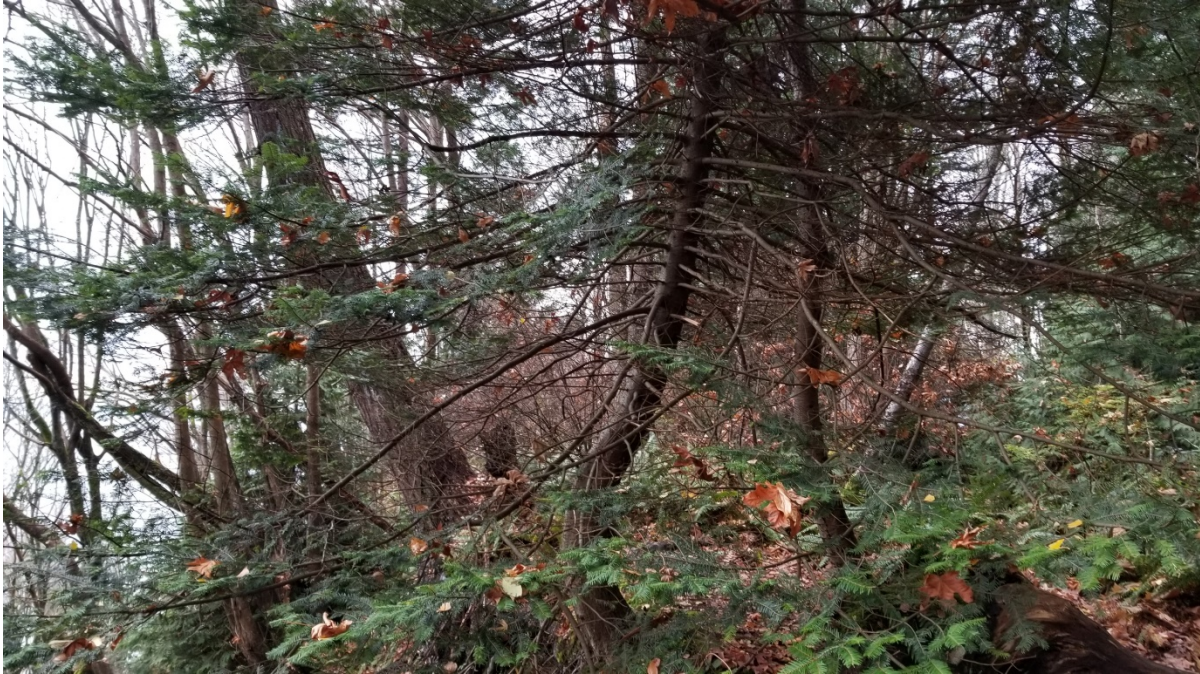
Picture taken at the edge of the cliff at Transect 1. The leaning trunks of the trees indicate gradual soil creep over the tree's growth.
