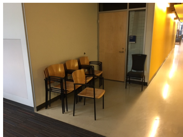
[4] Lack of storage throughout second floor. Code: Cluttered; Unwelcoming; Restrictive
