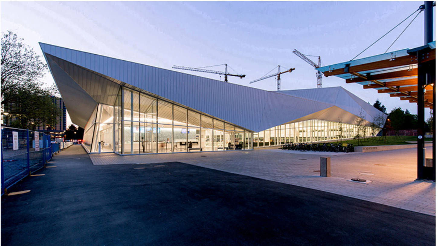
APPENDIX 2: EXERCISE PHOTOS - EXERCISE PHOTO 3. AQUATIC CENTER(HEATHERBRAE BUILDERS, 2016)
