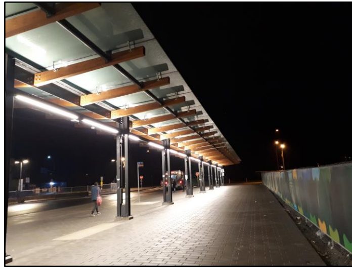
Figure 33: UBC 99 B-Line Bus Station Horizontal Overhead Covering and Well Lighted Physical Environment during Night Time
