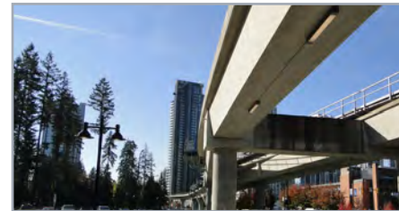
Lafarge-Lake Douglas guideways
