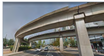
Curve guideway segment next to Science World Station
