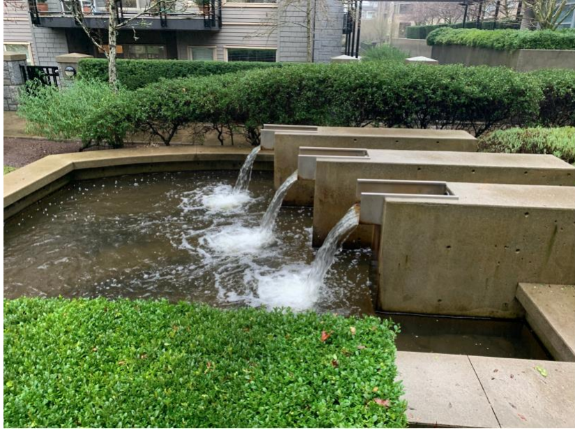
Figure 4. Fountains aerating stormwater in the channel at Khorana Park. [Photograph]. Emily Edwards.
