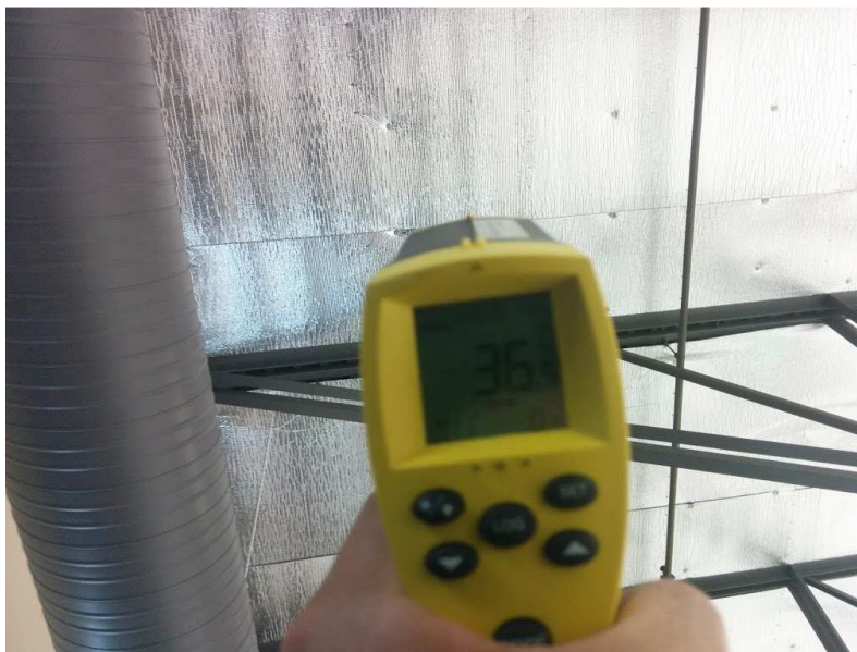
Figure 4 Reading 36.5°F (2.5 °C) of the low emissivity ceiling.
