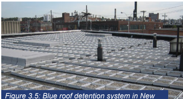
Figure 3.5: Blue roof detention system in New York City (The City of New York, 2016).
