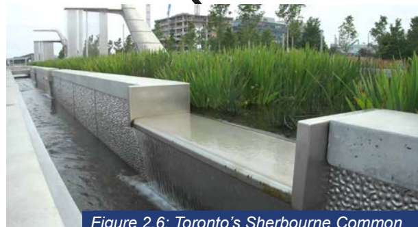
Figure 2.6: Toronto's Sherbourne Common stormwater channelling system (GBSS, 2014).
