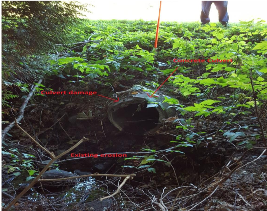
Figure 22 - Outflow Culvert at SW Marine DR and Wesbrook Mall
