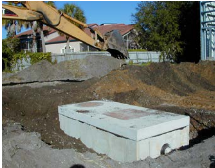
VortClarex™ installation in progress
