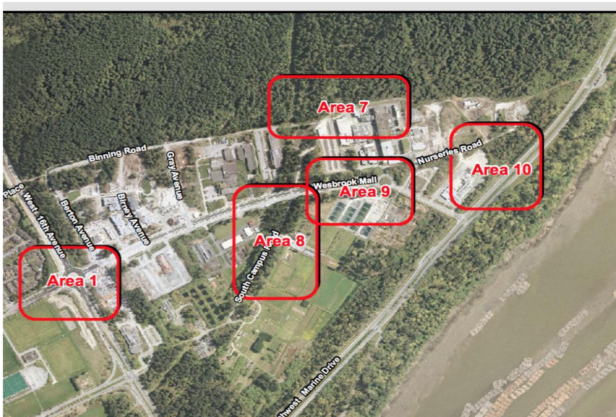
Figure 6: Overview of flood loss area in UBC South Campus
