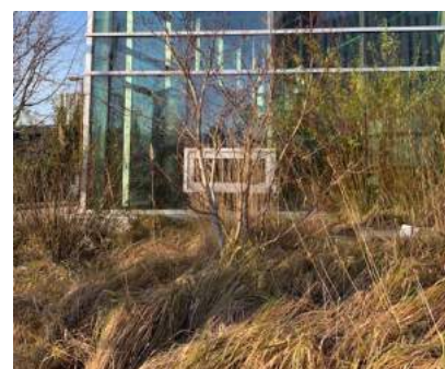
Figure 16. Lower slope condition
