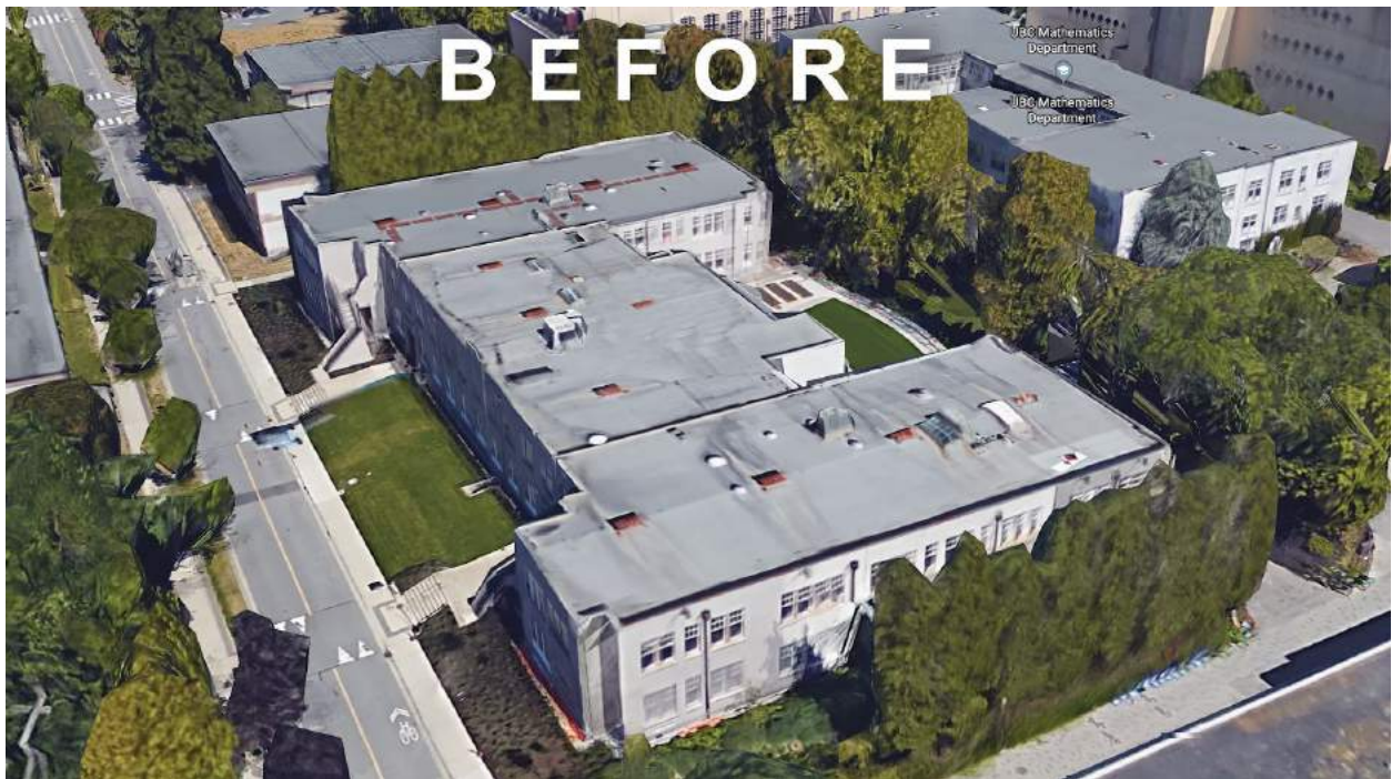
Figure 32: Before: Geography building roof
