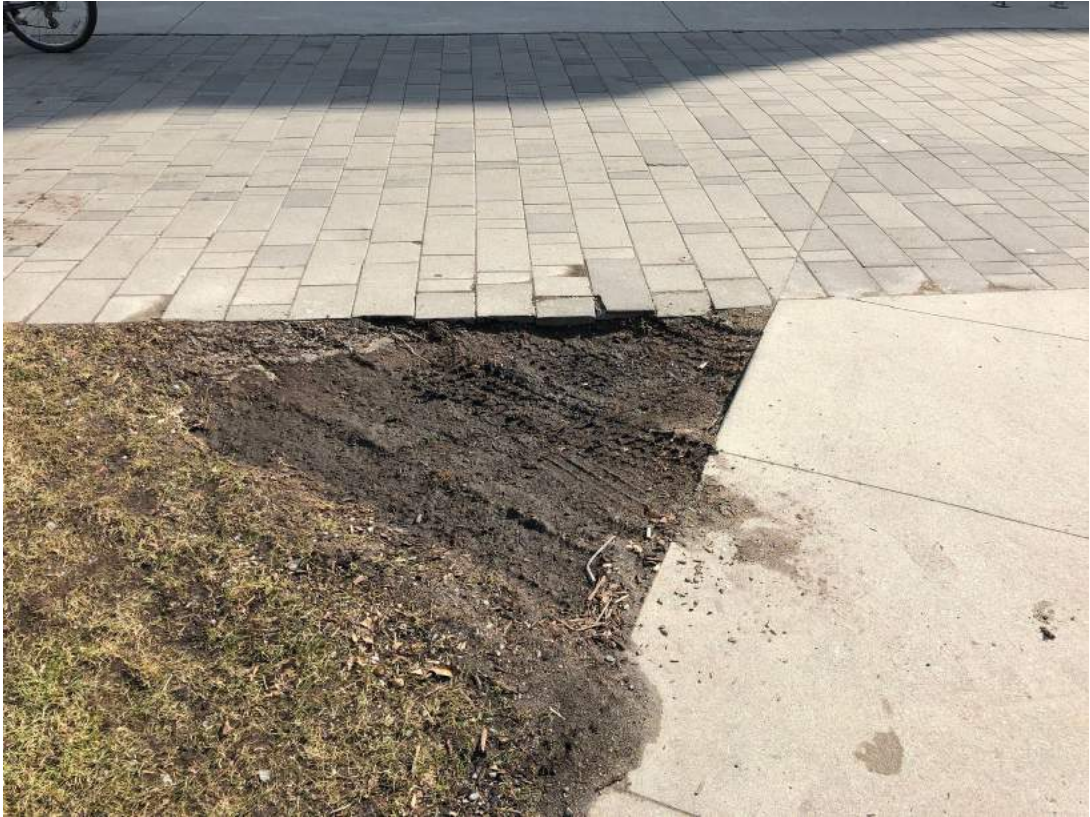
Figure 4: Soil compaction Zone 3
