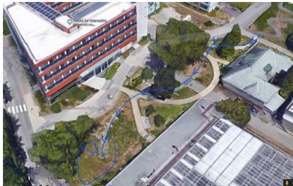
Figure 2. Google Map satellite picture for rainwater management system
