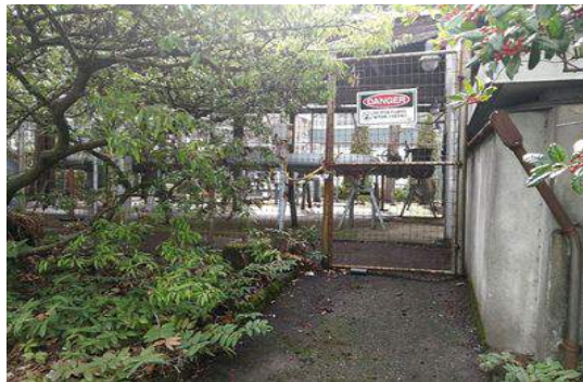
(Powerhouse in zone B)
