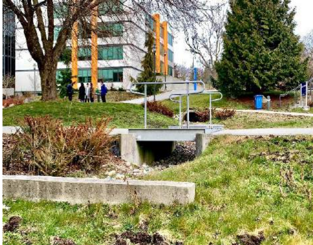
Figure 6. Open drainage channel
