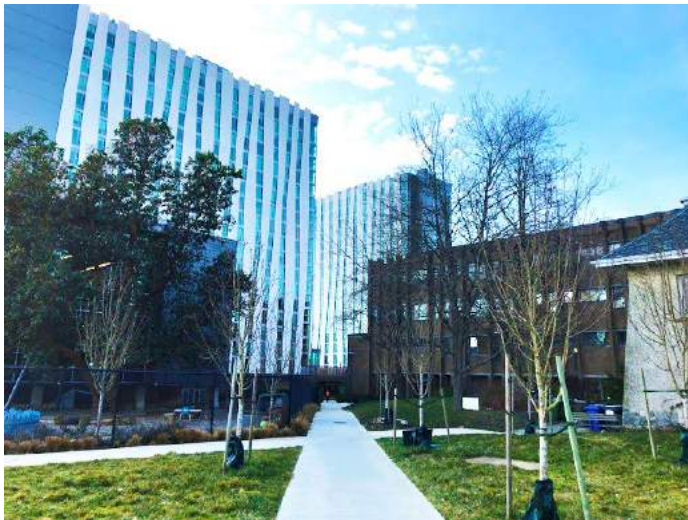
Figure 19. Subzone H: Pathway next to Orchard Commons and Daycare Centre
