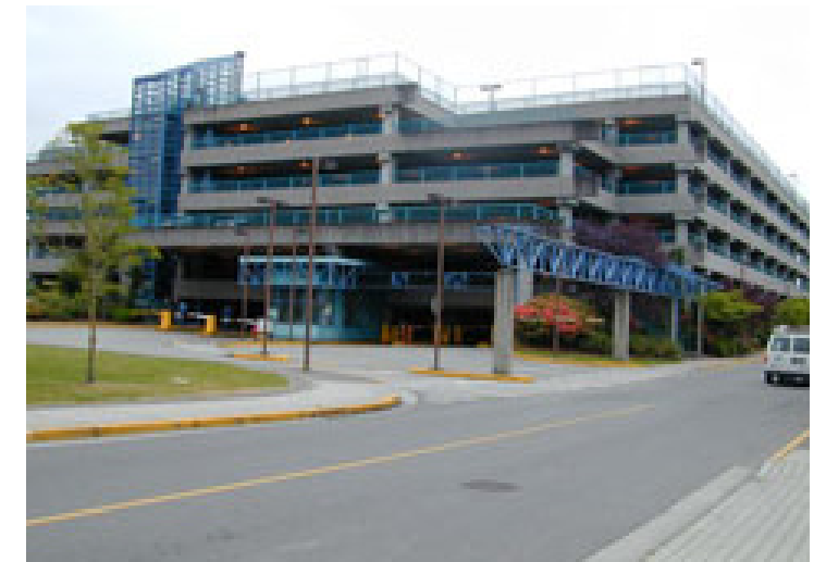
West Parkade, Above-Ground Structure
