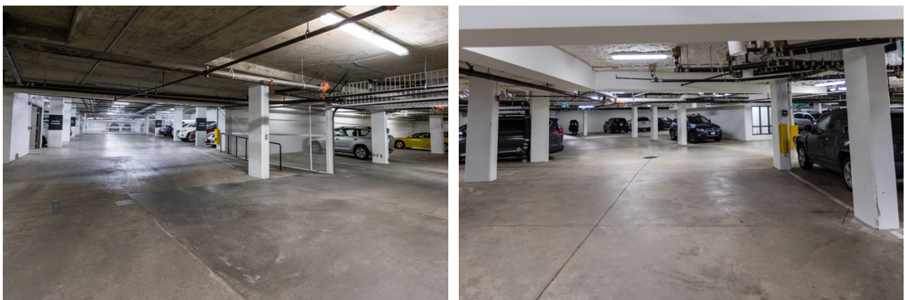
Figure 7.11: Cypress House - Condition of Cypress parkade, no dedicated pathway for bicycles
