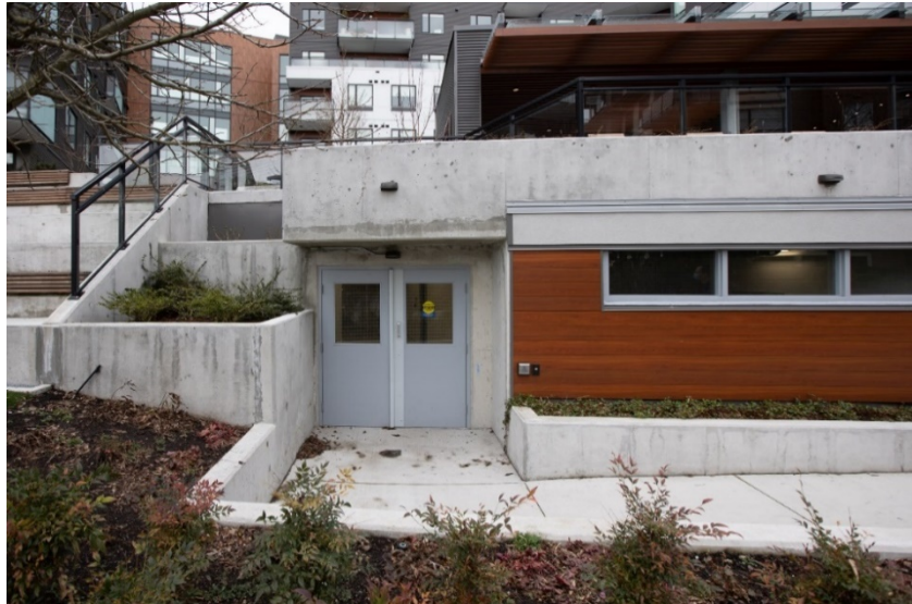
Automatic door at main entrance
