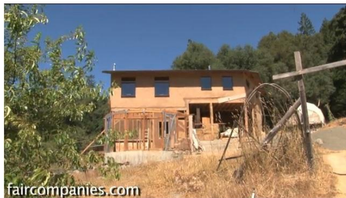
Figure 2: Emerald Earth Sanctuary Community Center located in Mendocino County California
