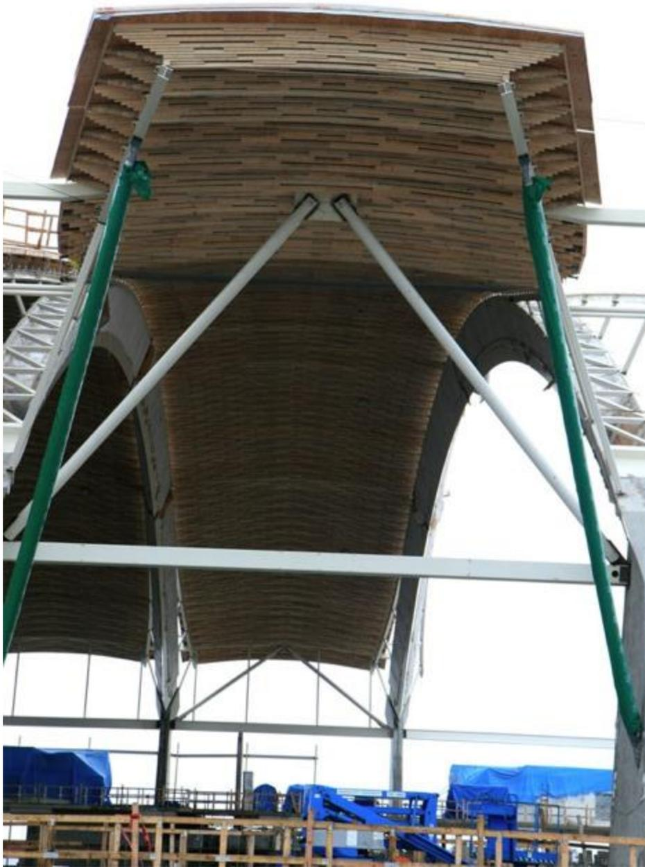
Figure 3 - Roof of Richmond Oval during construction
