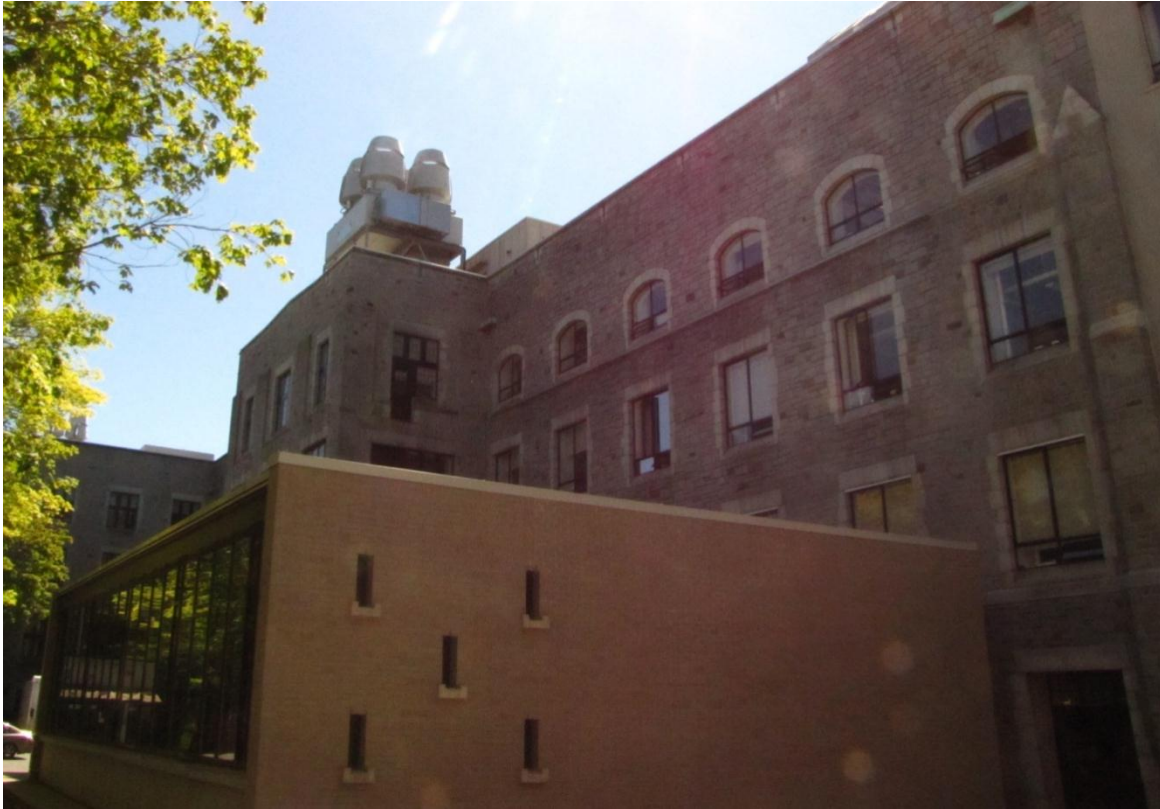
Figure 6 Rear view of CHEM D showing exhaust manifold and 4 HPE fans on the roof. The height of the 4 th level ceiling is visibly taller than the lower levels.
