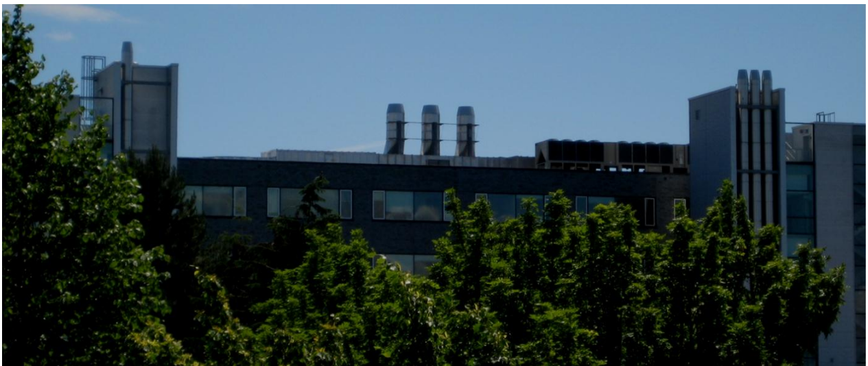
Figure 3 Exterior profile of the CHBE showing the 6 th floor and roof of the main tower. Exhaust stacks from the three wings are visible from left to right – one stack from the east wing, three HPE stacks from the main tower (connected to a sizeable exhaust manifold at their base), and three stacks from the CERC wing. The two chillers are visible between the two sets of triple-stacks.
