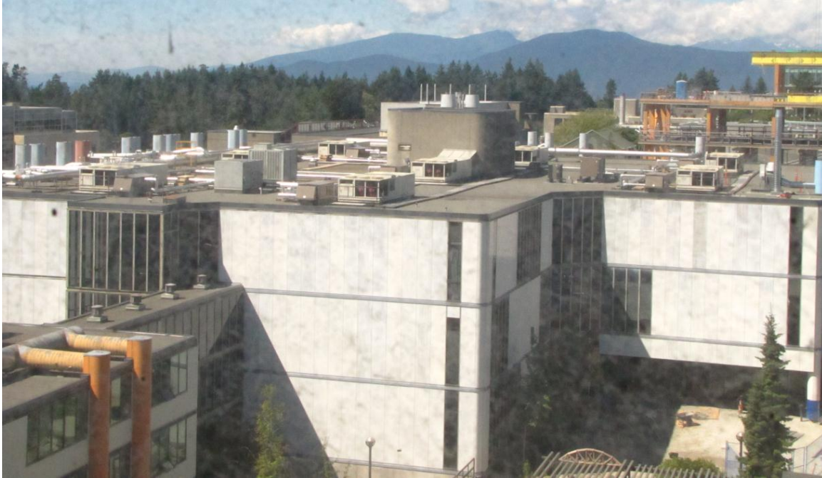
Figure 5 Exterior / roof level view of the EOSM building. Exhaust manifold is connected to two HPE fans, the tops of which are visible on the concrete enclosure at roof level.
