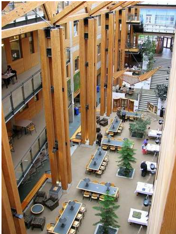
Figure 2: The L-shaped atrium that is a main attraction of the FSC. Source: flickr.com
